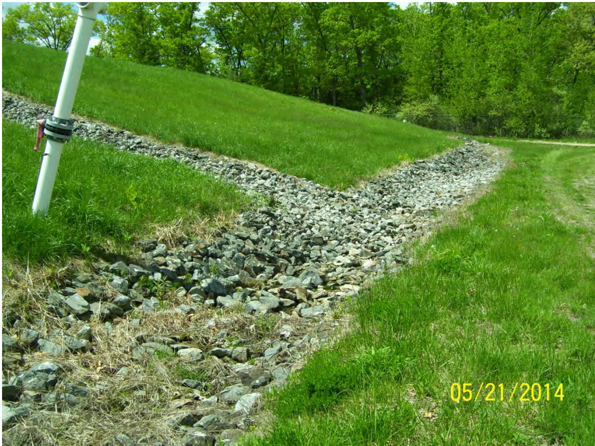
View of northwest bottom-of-slope drainage channel with minor vegetative growth
