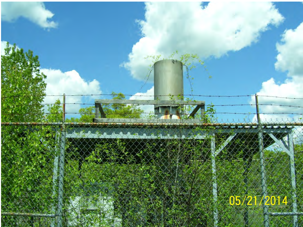
View of inactive thermal oxidizer unit stack
