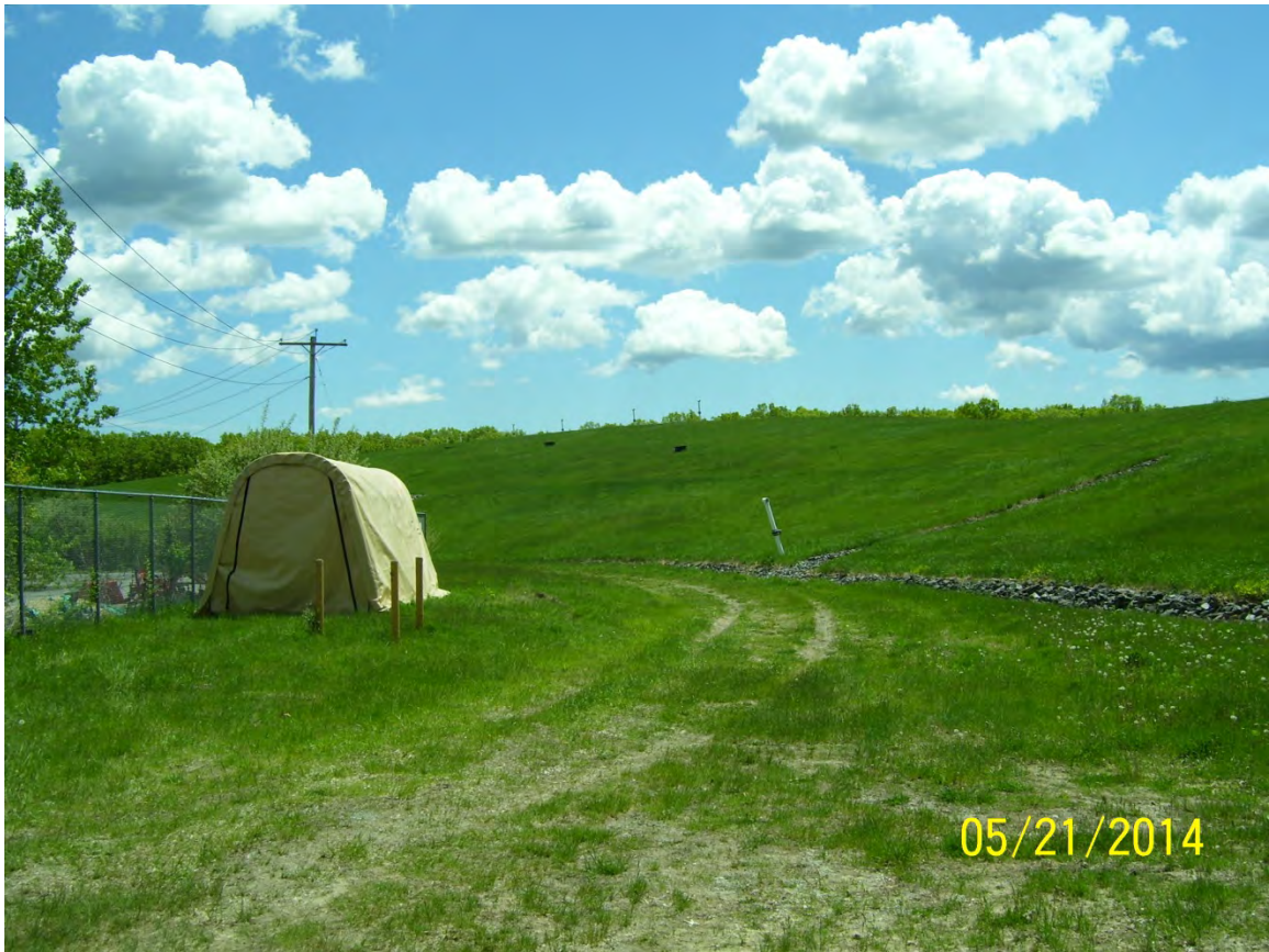
Northwest entrance of landfill, facing southeast
